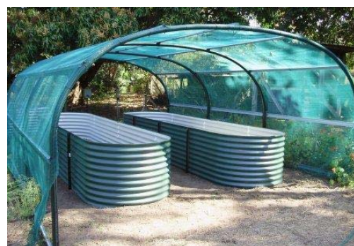
Photo 12, still under construction
